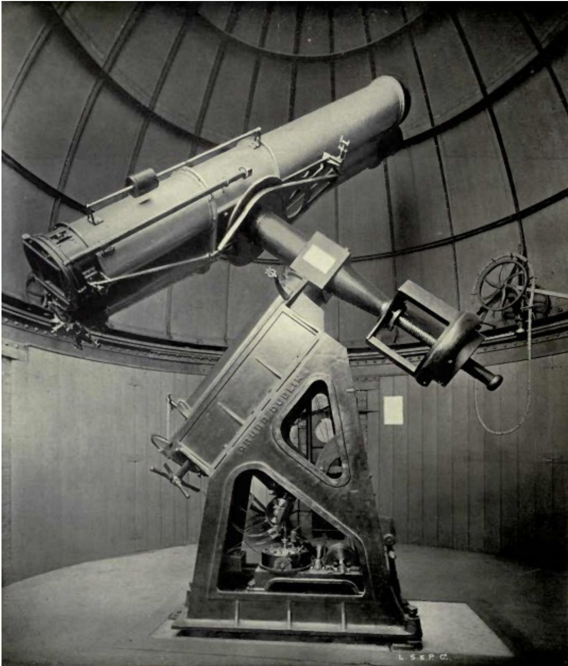
Greenwich Observatory Astrograph, built by Sir Howard Grubb, c1891
